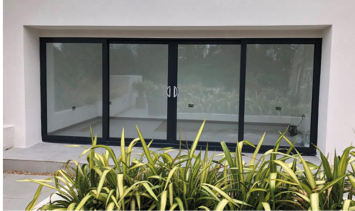
All glass units are made from heat treated toughened safety glass, to offer safety and to comply with modern building regulations.
